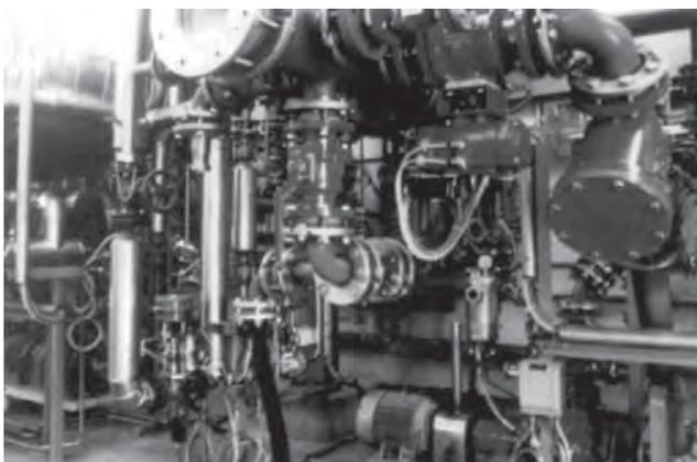
Fig. 1: Fluoropolymer lined valves in a chemical plant.
