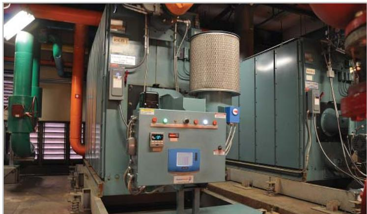
The new CB ProFire MTH Burner and control panel on one of the boilers
