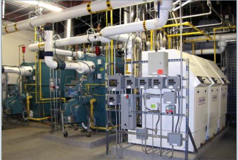
An integrated control system accounts for an array of operating factors to automatically control the firing of boilers in a complete system
