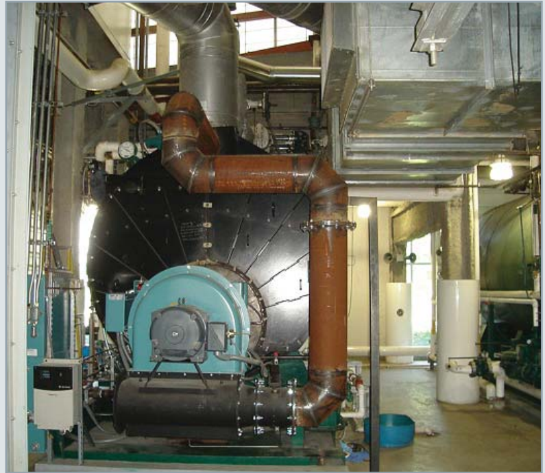
Final retrofit in the UC Davis Medical Center
