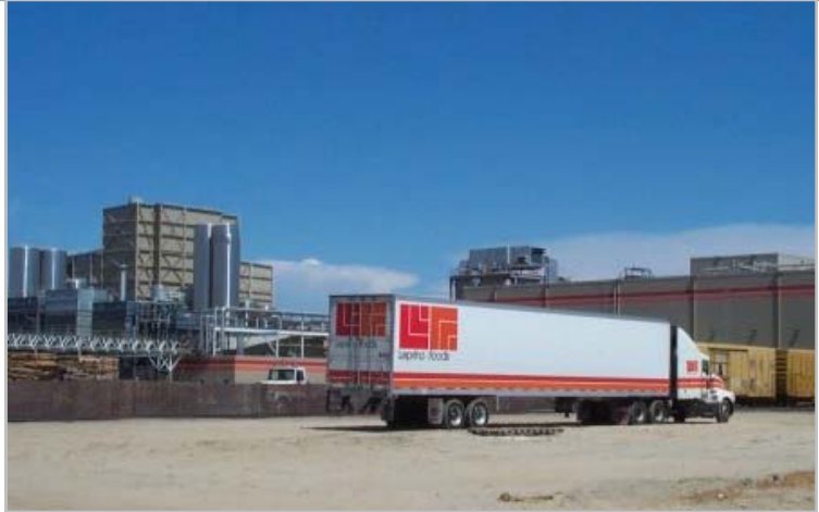
The Leprino Foods Lemoore West facility
