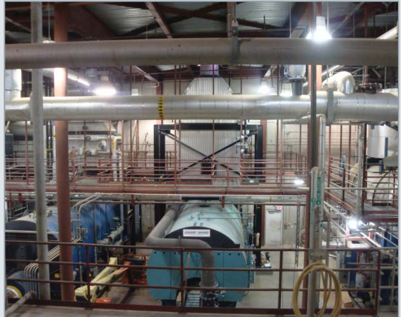
Final installation of Boiler and SCR system
