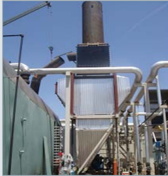
Installation of the new SCR and flue stack
