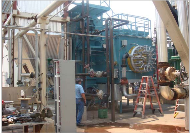
Field service technician commissioning the new burner/scr system
