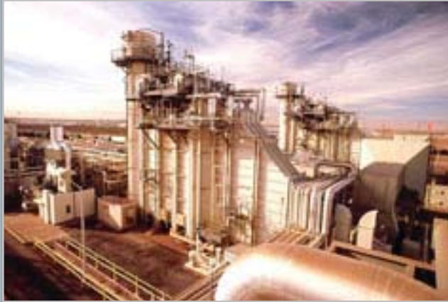
The Saguaro Power Company in Henderson, Nevada
