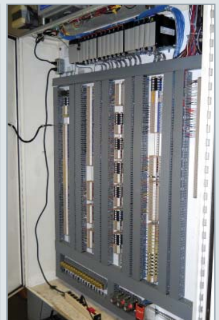
The Burner Management System Panel (BMS) - Before on Left and After on the Right
