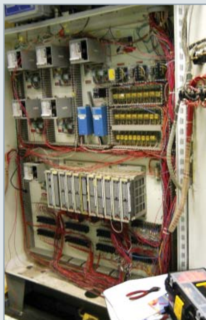
The Burner Management System Panel (BMS) - Before on Left and After on the Right
