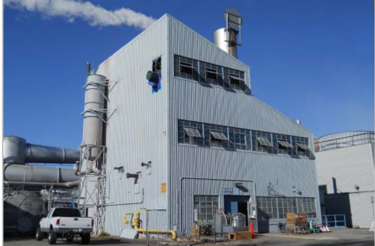
The Arc Jet Complex at NASA houses the three story boiler and new controls
