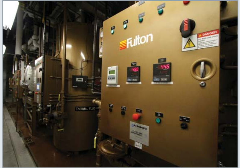
Final installation of Fulton Thermal Fluid Systems
