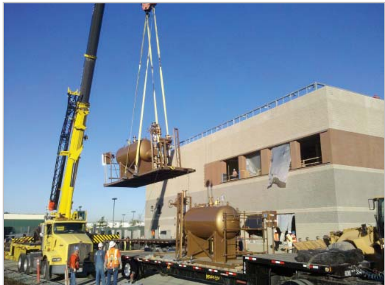
Fully loaded skids delivered through the 10'x12' third floor louver openings
